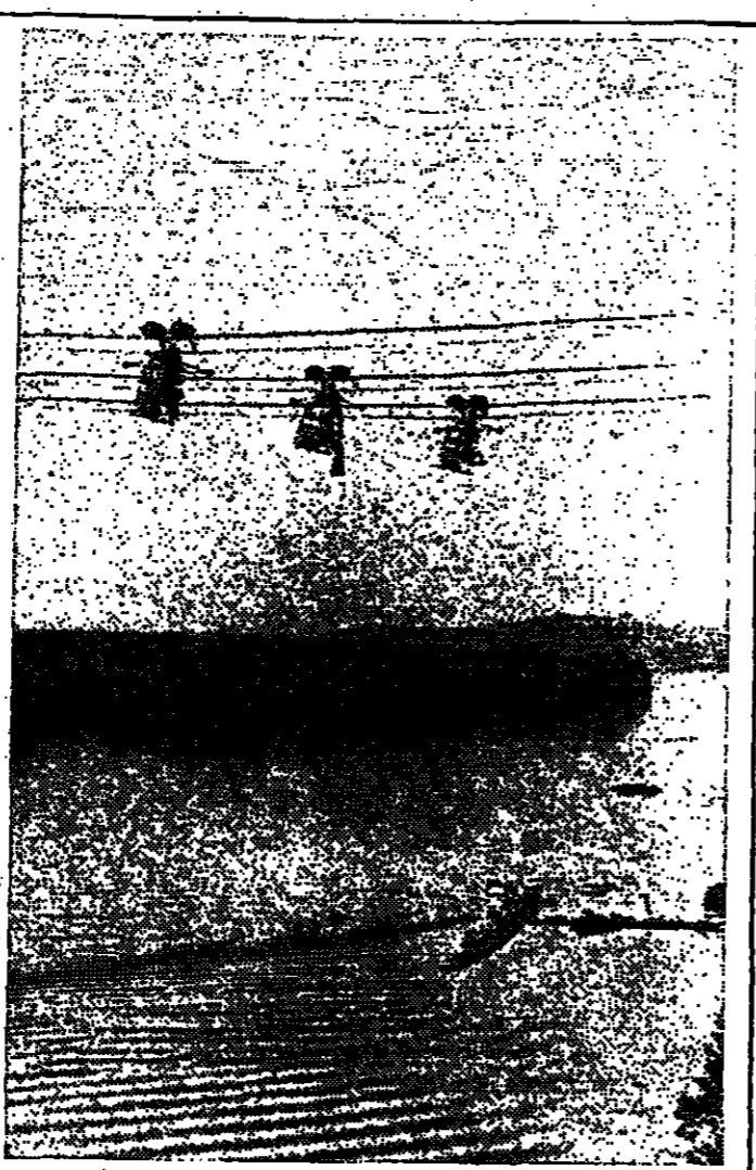
HIGH POWER—Electric linemen riding gasoline powered carts inspecting and making final adjustments on Niagara Mohawk's 765,000-volt transmission line.
